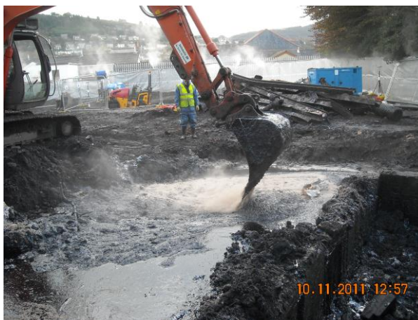
Figure 2. Remediation at Briton Ferry Gas Works
