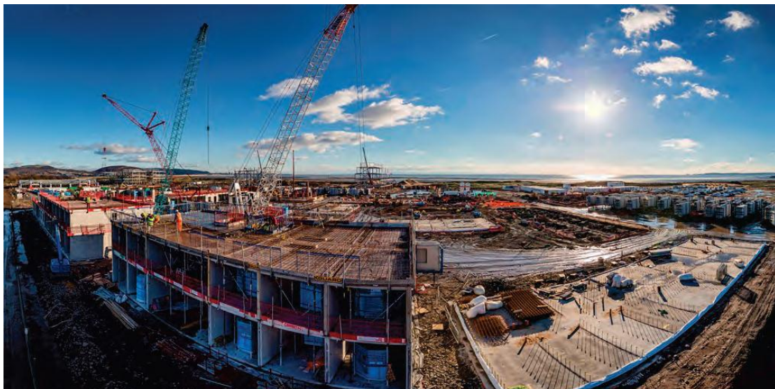
Figure 8. Swansea University Campus under construction
